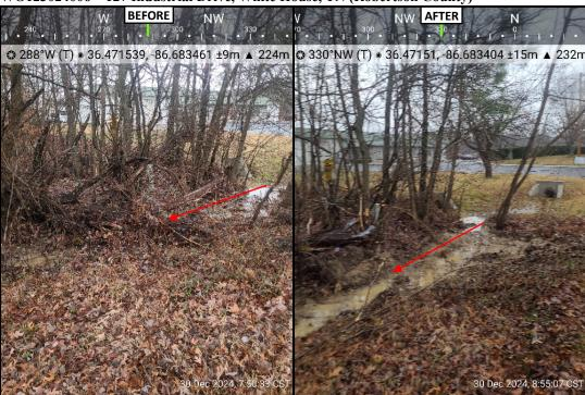
Notes: We received a called about flooding. Upon inspection, a tree was blocking the area. The tree was removed to provide positive flow.
