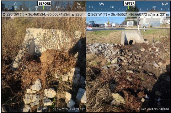
Notes: Pine needles from upgradient pine trees clogged up the drainage pipe and required clean out.
