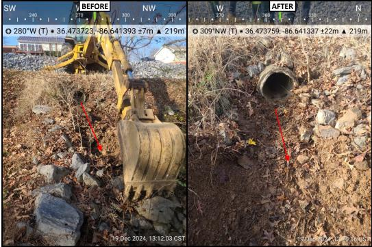
Notes: Received homeowner complaint regarding drainage issues. We reshaped outlet to provide direct drainage to stream.
