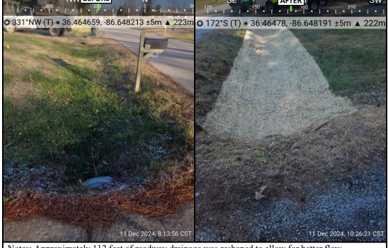
Notes: Approximately 112 feet of roadway drainage was reshaped to allow for better flow.
