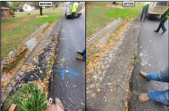
Notes: We repaired this area, but the hurricane came in and washed out the drainage. We repaired the system again by the road. The flex matting is work great.
