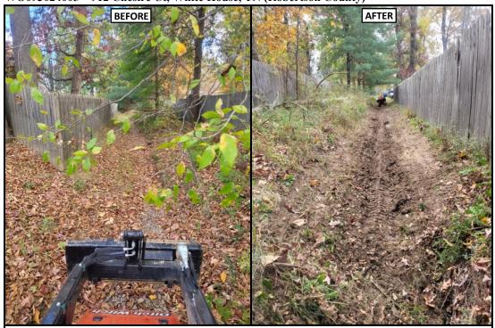
Notes: We cleaned out the brush and build-up in the drainage system to help with the flooding in this area.
