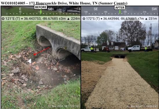
Notes: The area by the outfall was full of buildup and was causing backup. We cleaned the area and used the dirt to repair the area that washed out during the storms.
