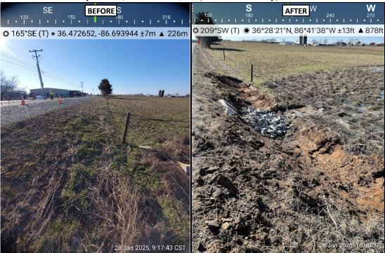
Notes: The Division cleaned out the drainage off of Pleasant Grove Road and added a new ditch line to allow positive stormwater flow.
