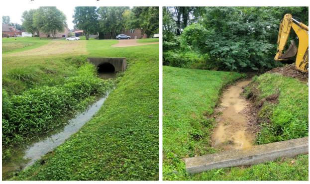
**524 North Palmers Chapel** – Repaired sinkhole in driveway with new material. These culverts will need total replacement for long-term functionality.
