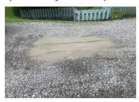
108 Louise - Removed clogged pipe and built a berm to help channel water to ditch.
